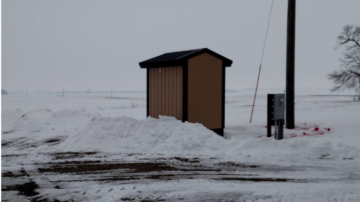
Figure 5 Looking at the existing wellhouse
