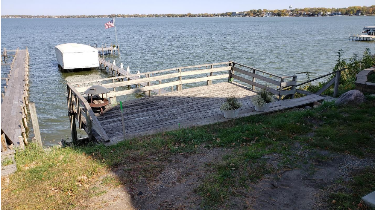
Figure 1 Looking at the existing deck
