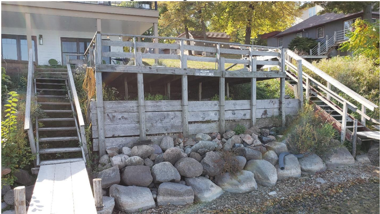
Figure 2 Looking at the existing deck built into the bank
