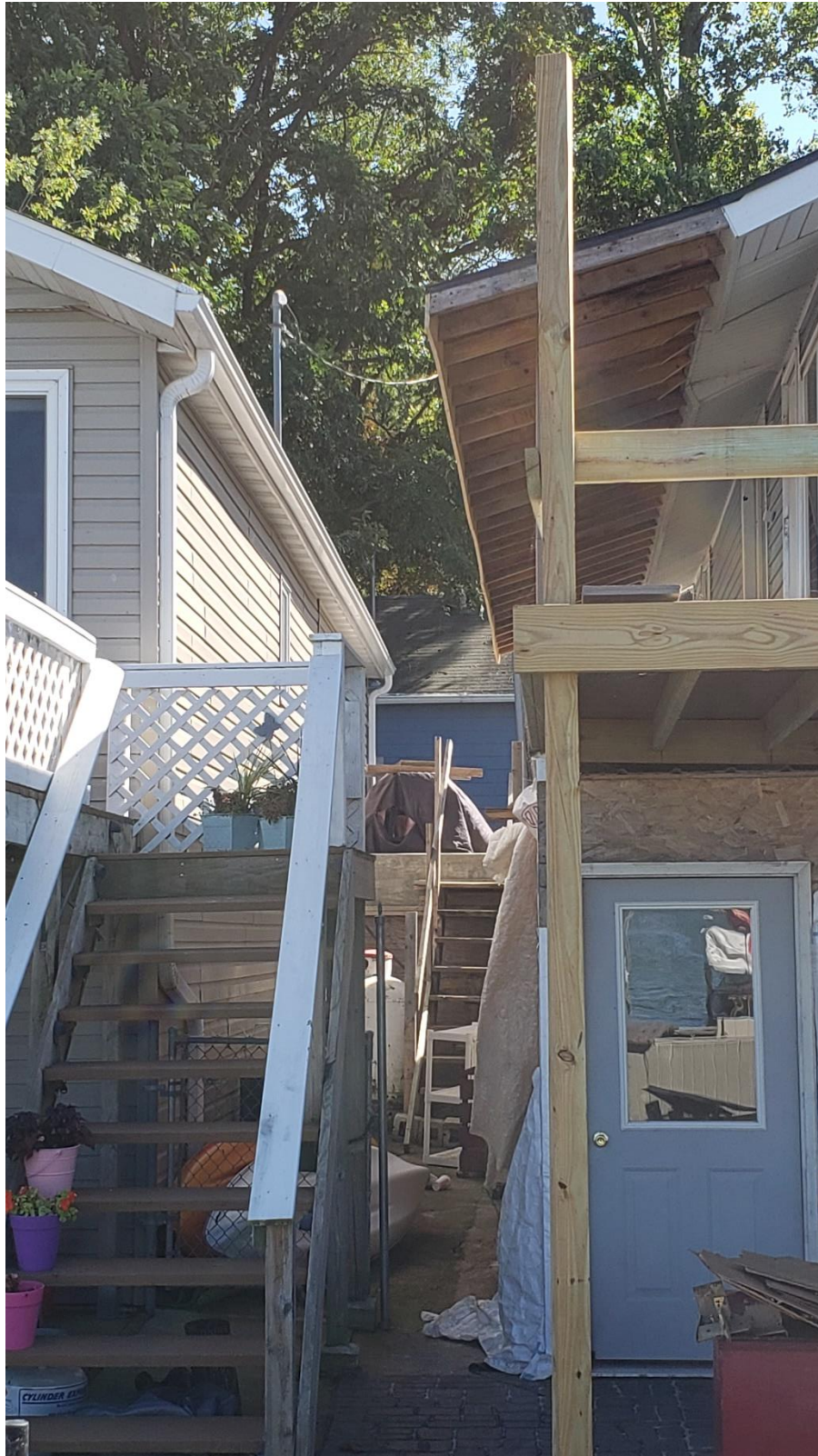
Figure 4 Looking south along the east side lot line
