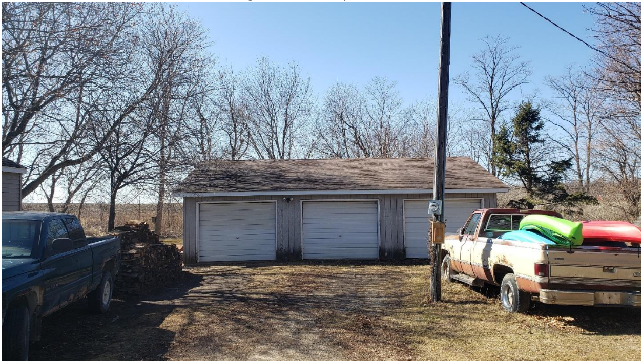
Figure 4 Looking at the westerly machine shed
