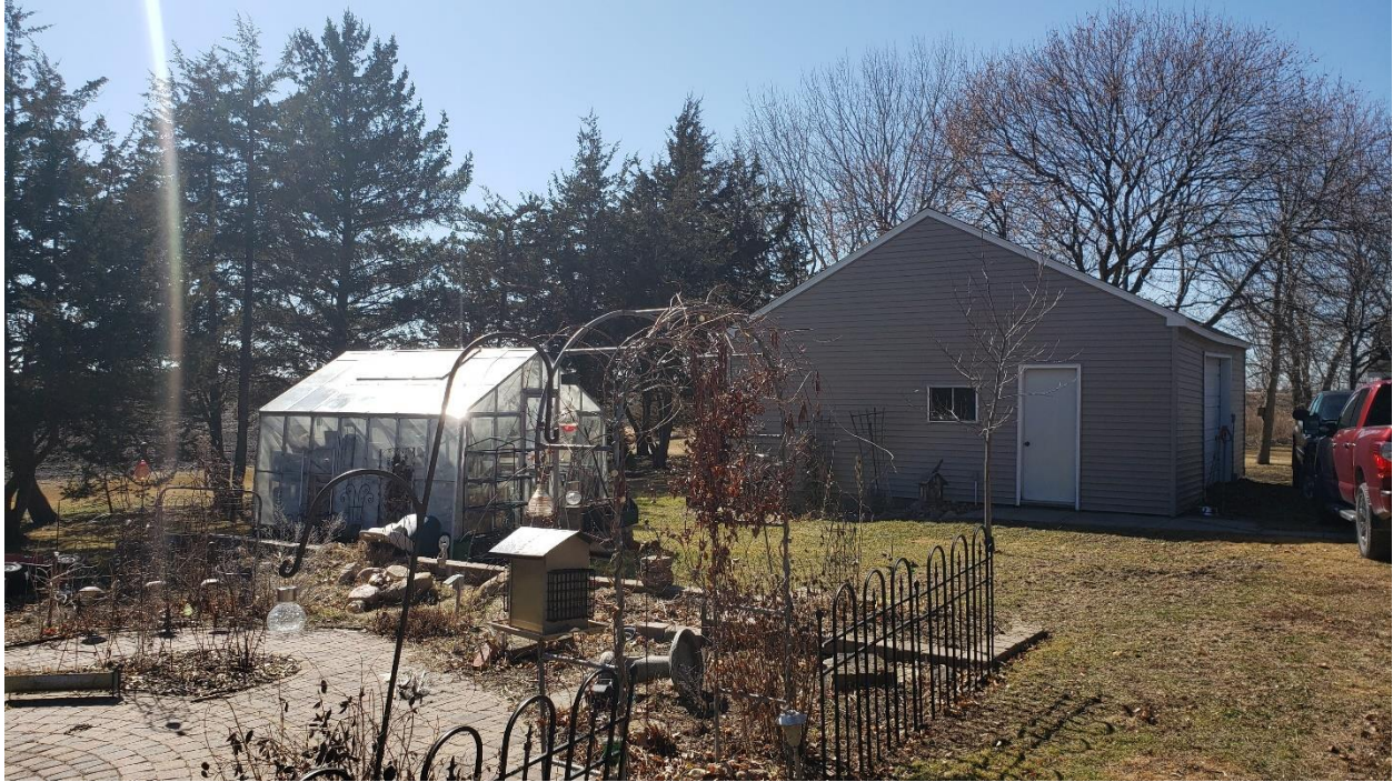
Figure 3 Looking at the southerly garden shed and machine shed
