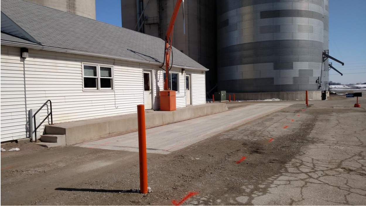
Figure 3 Looking at the existing truck scale
