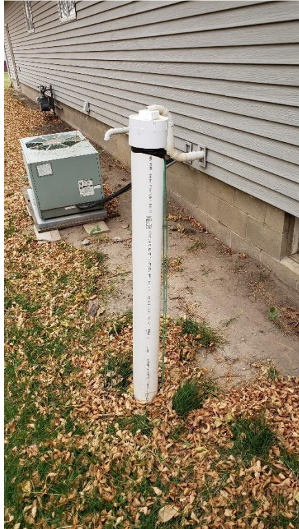
Figure 7 Looking at the existing well
