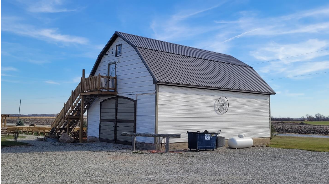
Figure 5 Looking at the converted corn crib
