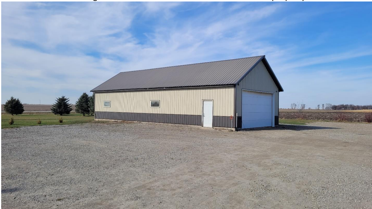
Figure 6 Looking at the machine shed at the north side of the property
