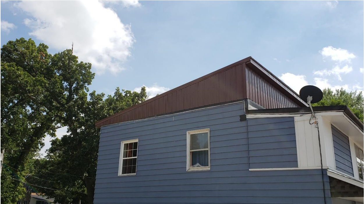
Figure 1 Looking at the added pitched roof
