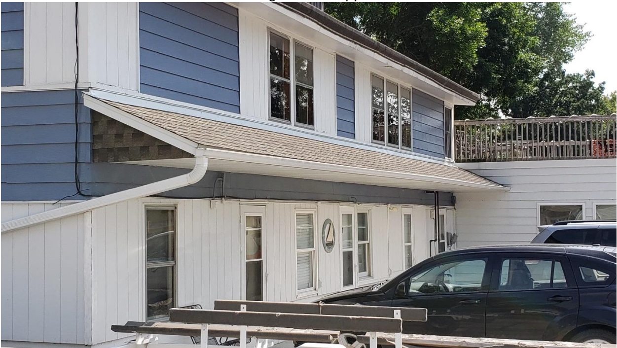
Figure 2 Looking at the canopy roof
